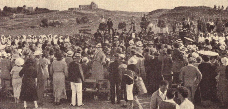
Laying of Cornerstone for Hadassah-University Hospital on Mt. Scopus, (J.N.F. Site)
